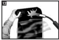
Partially remove the release liner and gently heat the underlap approximately 150 mm (6") from the
